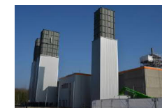
Combustion Test Center in Berlin
