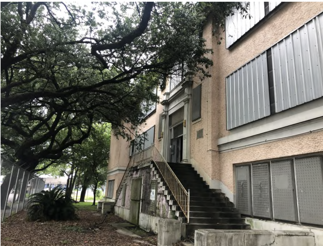
Facade in 2019, before brownfield assessments began.
