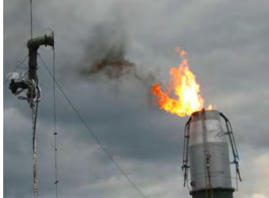
Photo: Air-Assisted Flare Measured at 99.4% Efficiency
