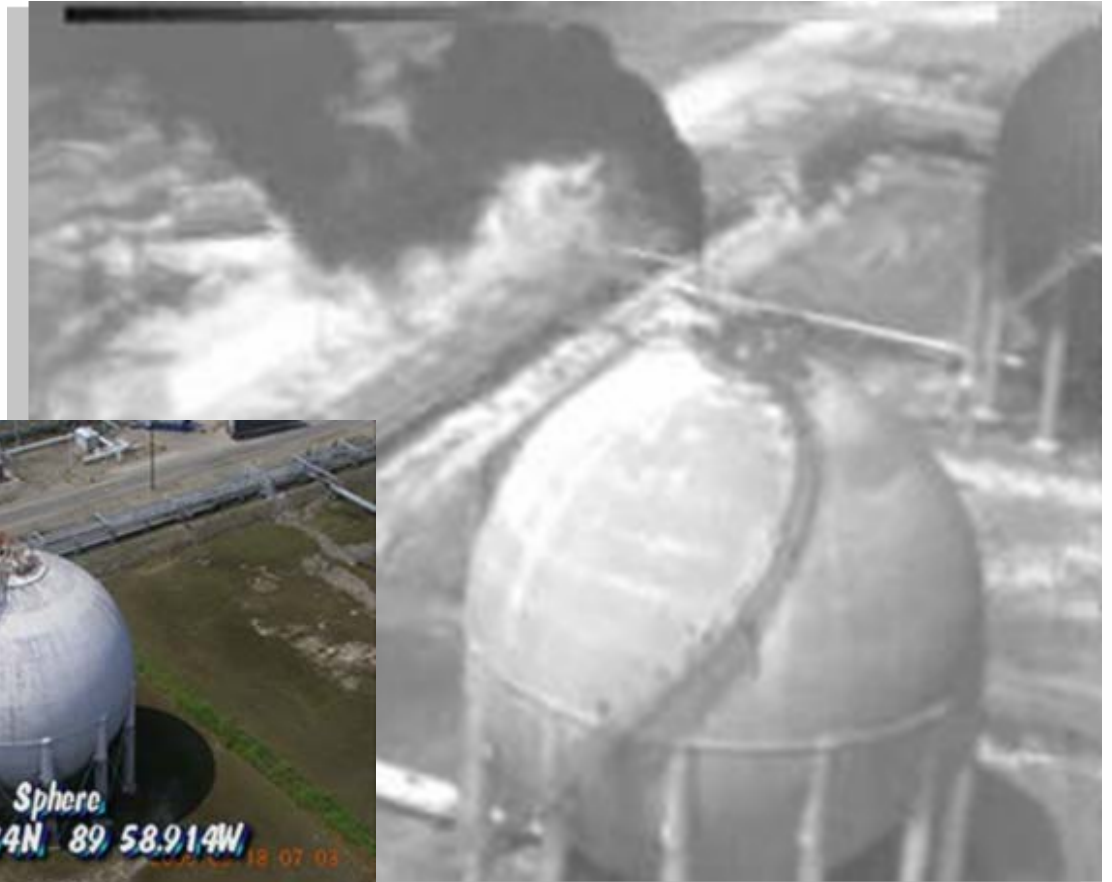
HAWK Image of Leaking Propane Sphere
