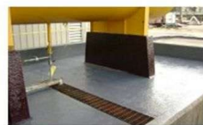
Belzona 4311 (Magma CR1) Epoxy novolac, high chemical-resistant barrier coating for concrete and steel protection.
