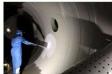
Belzona 5892 Epoxy barrier coating suitable for surfaces in contact with aqueous solutions at temperatures up to 95^{\circ}\text{C} ( 203^{\circ}\text{F} ).
