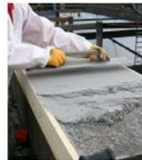
Belzona 4131 (Magma-Screed) Epoxy impact and abrasion-resistant concrete repair mortar.
