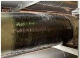
Belzona 1983 High temperature resin for application temperatures of 5°C (41°F) - 40°C (104°F) and operating temperatures up to 150°C (302°F).
