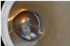
Belzona 1381 Sprayable, erosion-corrosion resistant epoxy coating with ultra high molecular weight polymer fillers for immersion up to 95^{\circ}\text{C} ( 203^{\circ}\text{F} ).
