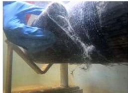
Belzona 1984 Surface tolerant resin for service temperatures up to 50°C (122°F) and suitable for minimum application temperature of 5°C (41°F).
