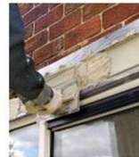
Belzona 4141 (Magma-Build) Lightweight epoxy concrete repair mortar suitable for vertical and overhead applications.
