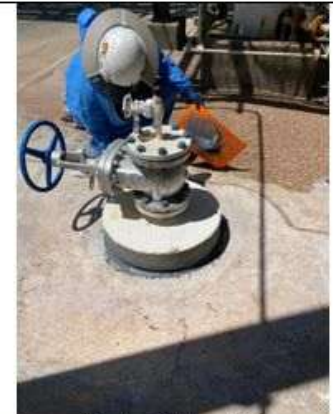
Chamfer with Belzona 1121
