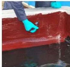
Belzona 4361 Flexible chemical resistant epoxy barrier coating suitable for concrete protection. Particularly suitable for areas subject to movement.
