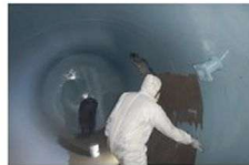
Belzona 1391T Hand-applied, high-temperature, abrasion-resistant epoxy coating for erosion-corrosion protection under immersion up to 130^{\circ}\text{C} ( 266^{\circ}\text{F} ).
