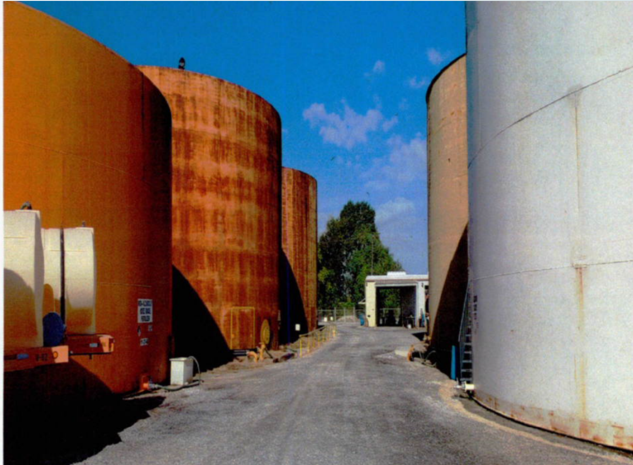
Photo #: 1 of 8 Date: 9/24/2024 Time: 9:30 AM Description: Layout of the first corridor of large tanks towards the front of the facility. Tanks holding multiple chemicals. No containment seen around these tanks.
